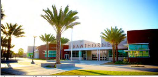
Hawthorne HS Administration Bldg.
